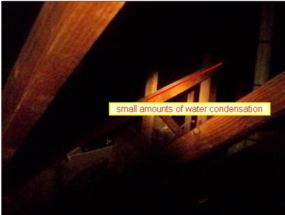
1.5 Picture 3 roof structure and attic
